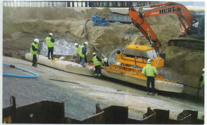
Figure 5 above left: The 3.2km toe beam under construction.
