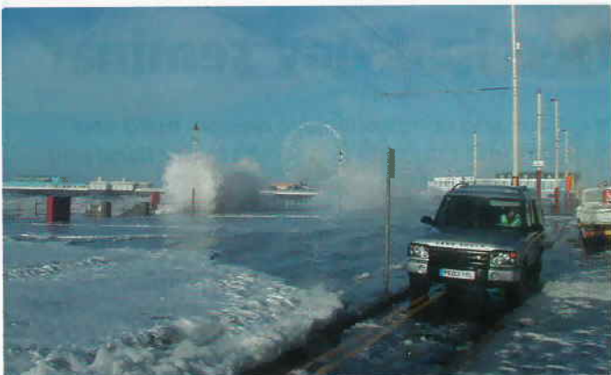
Figure 1 above: Marine defence work aims to protect 1500 at-risk properties from similar flooding.
