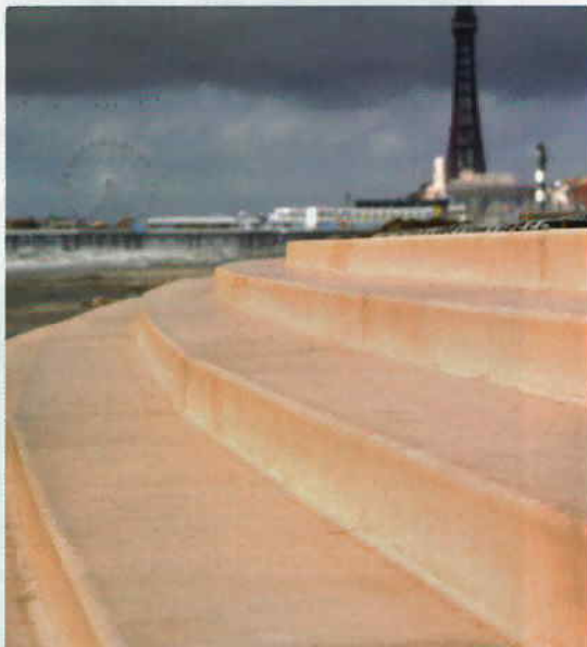
Figures 2 and 3: The completed seafront scheme.
