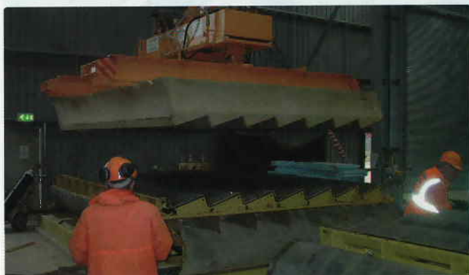
Figure 4 below right: Load testing the revetment units.
