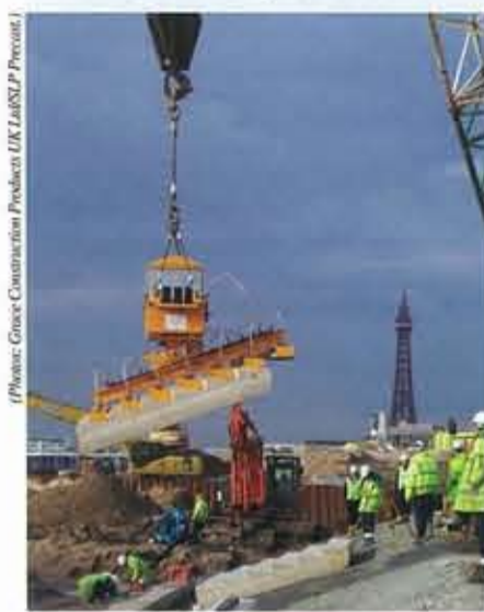
Figure 1: Vacuum machine lowering precast unit in front of toe beam.
