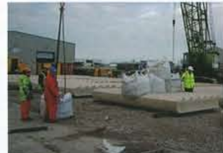
Figure 3: Load testing of the revetment units.
