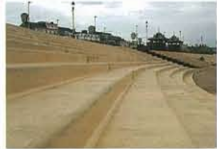
Figure 4: Some of the first revetment units in place.
